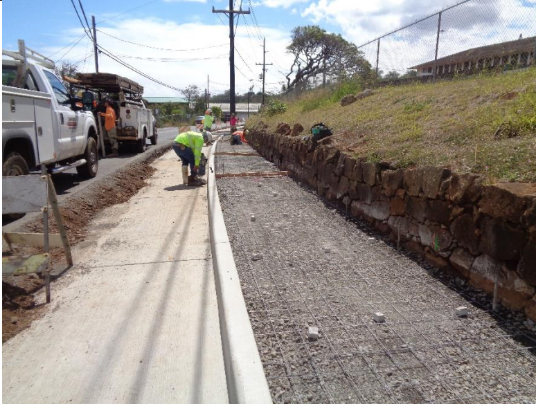
DSC03179 Placed WWM for sidewalk.
