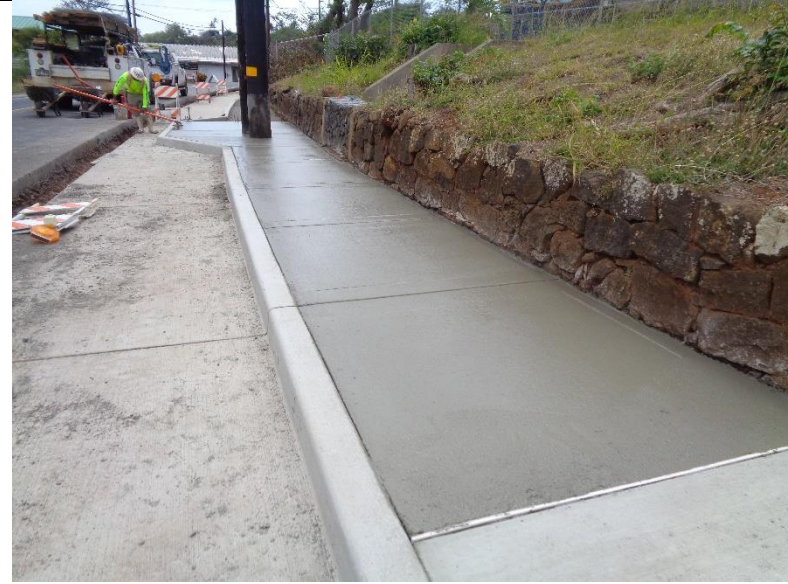
DSC03213 Freshly poured and finished concrete sidewalk.
