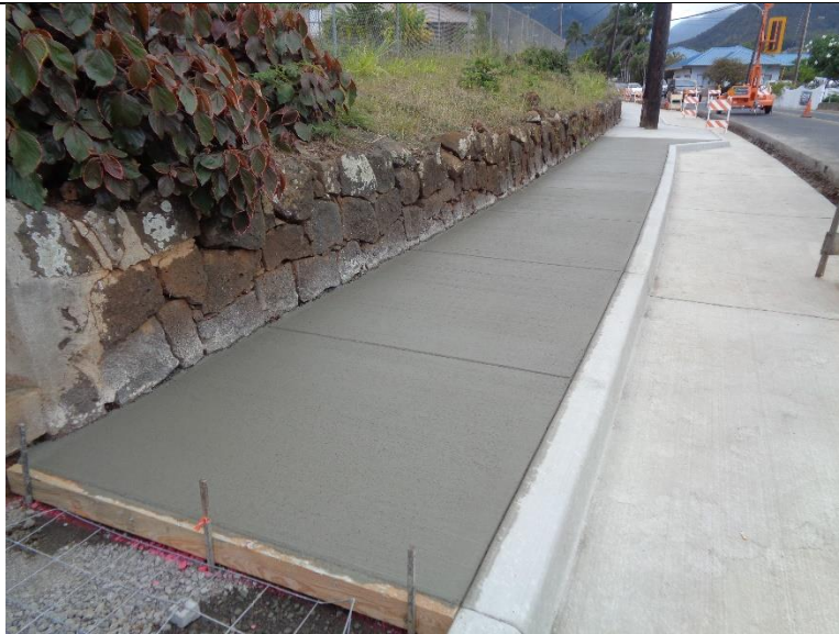
DSC03296 Freshly poured and finished concrete sidewalk
