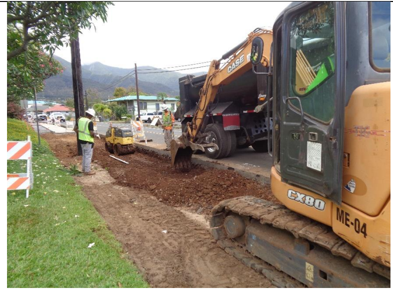
DSC03295 Excavation for curb and gutter swale.
