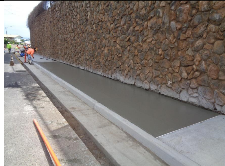
DSC02344 Poured concrete sidewalk at Mill St
