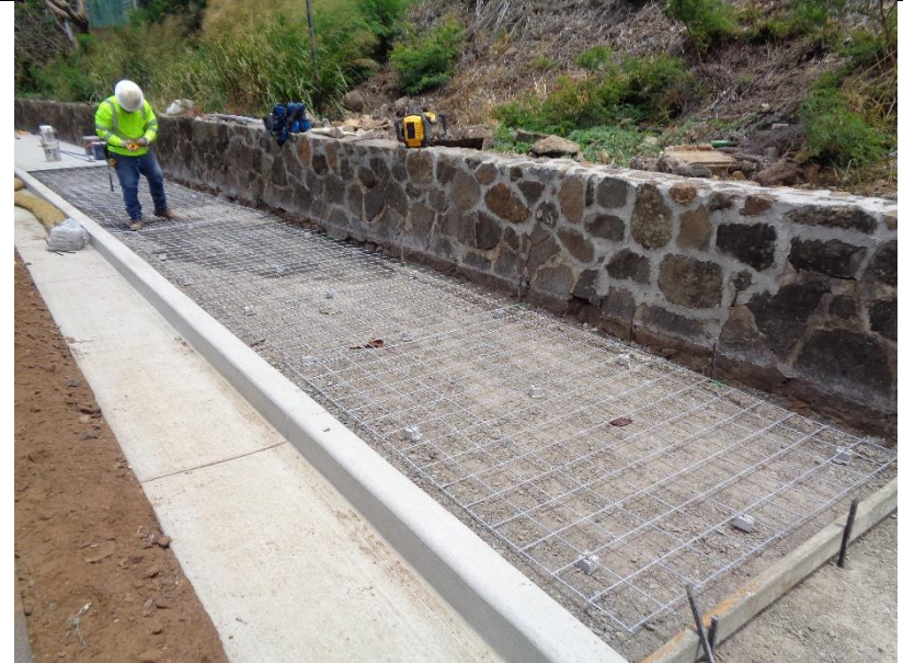
DSC02350 – Prep sidewalk subgrade
