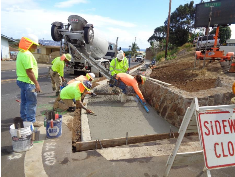
DSC02363 – Pouring concrete sidewalk at Mill St and Olu Dr.
