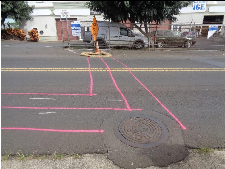
DSC02338 Layout drainline.
