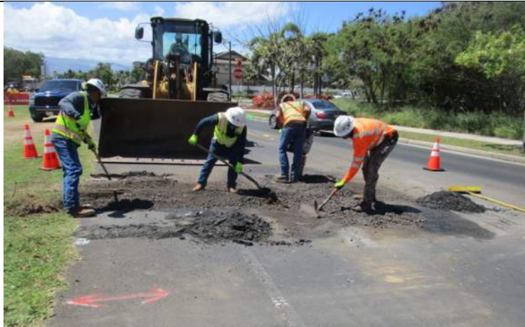
Place UTB for fire hydrant lateral trench excavation.
