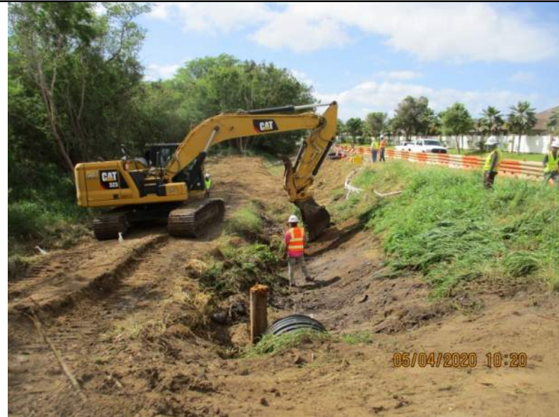
Grubbing location of new 48-inch HDPE drainline alignment.
