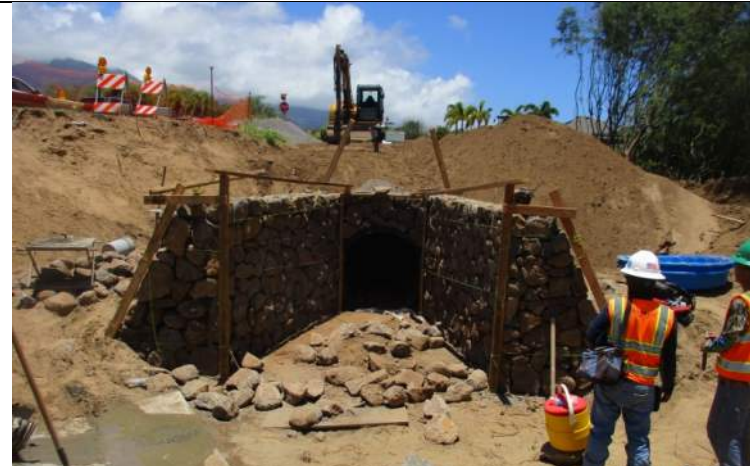
Completed CRM drainline outlet headwall.
