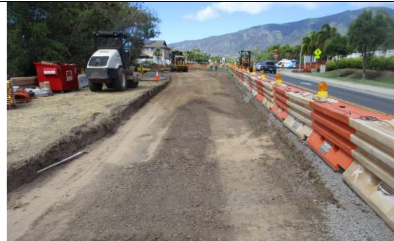
Sub-grade prep for new roadway along Kamehameha Avenue.
