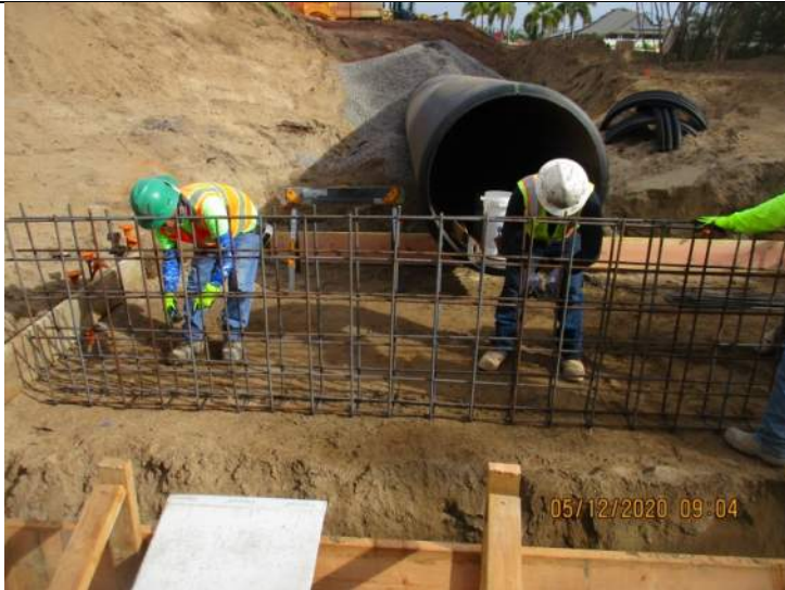
Fabricating reinforcing steel for the drainline outlet slab cutoff wall.
