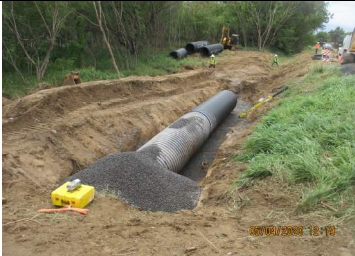
Portion of new 48-inch HDPE drainline.
