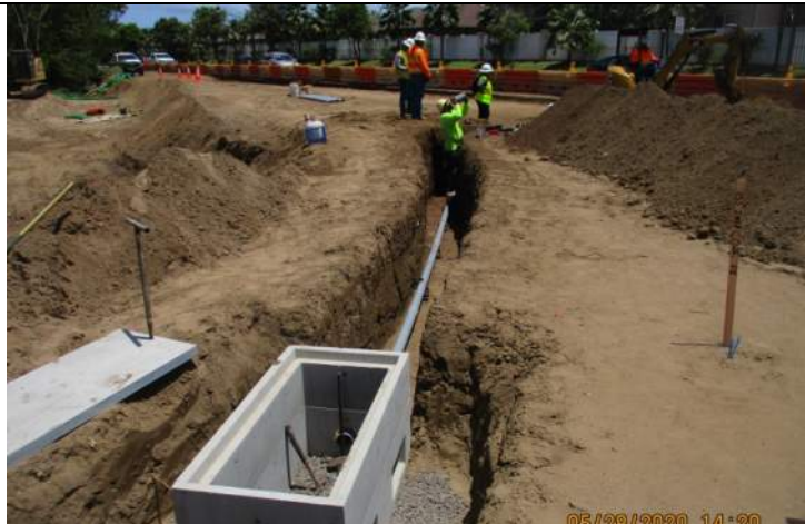
New 2-inch PVC Schedule 40 electrical conduit ductline installation.
